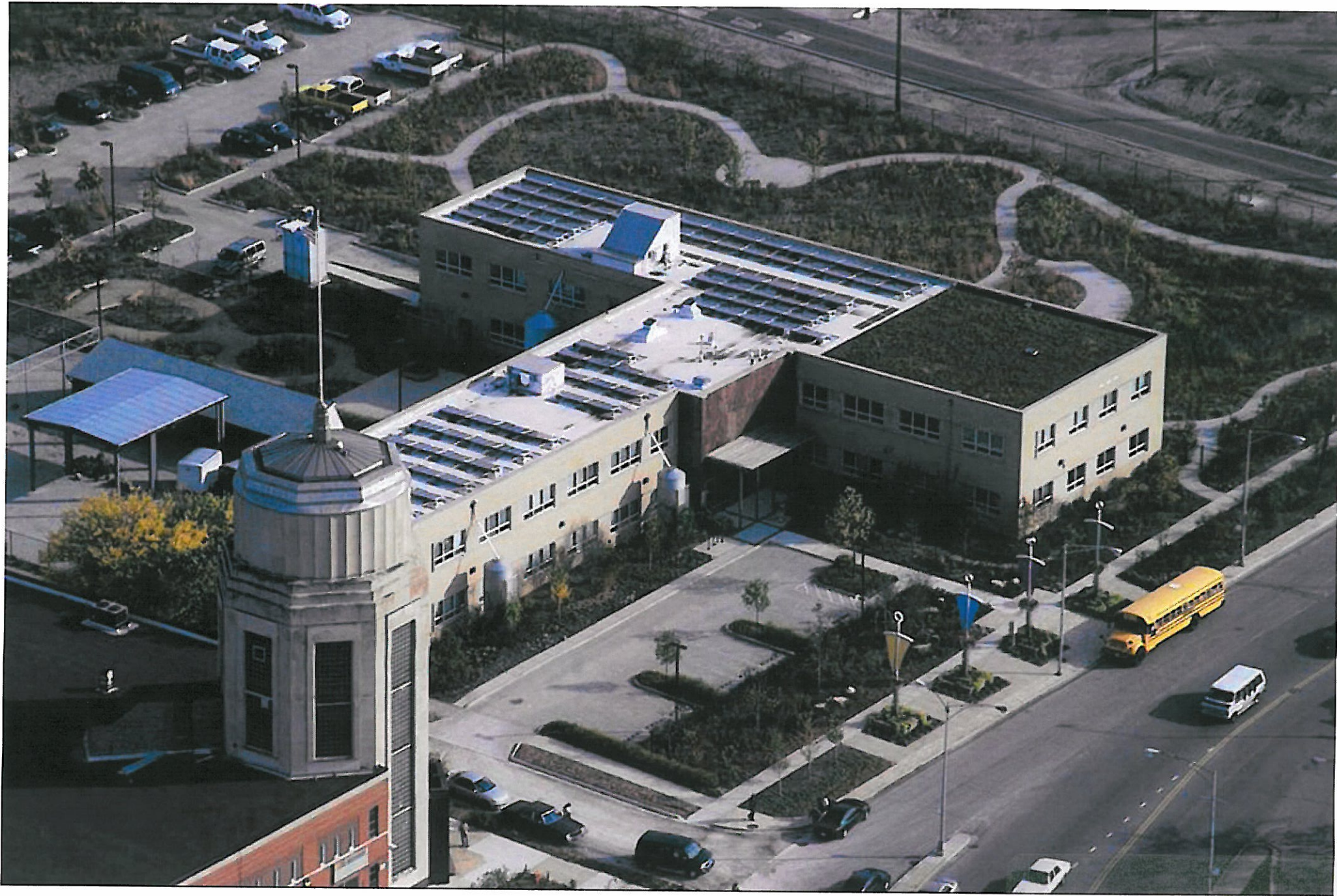
Chicago Center for Green Technology - SITE Design Group
