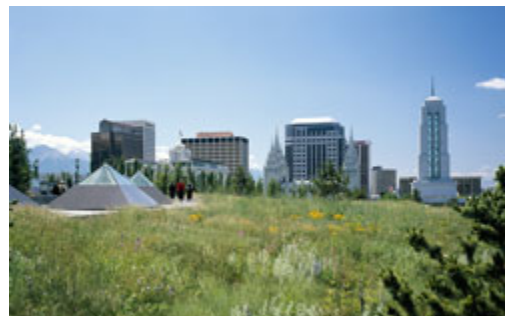
Figure 10. The Church of Jesus Christ of Latter-Day Saints Convention Center. Courtesy Green Roofs for Healthy Cities) and Olin Partnership
