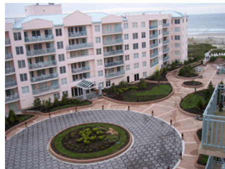
Figure 4. Seapointe Village Deck Restoration. Courtesy Green Roofs for Healthy Cities and Jeffrey L. Bruce & Co.
