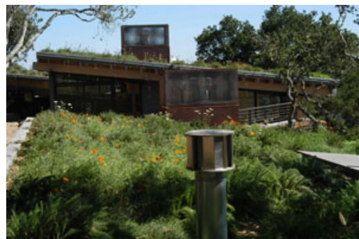
Figure 12. Feldman Residence. Courtesy Green Roofs for Healthy Cities and Rana Creek.
