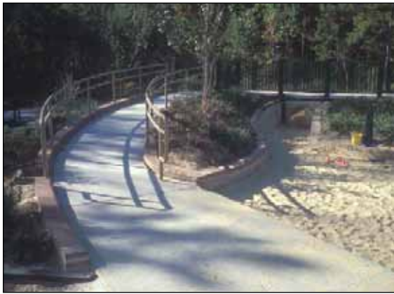
Figure 36. A ramp over a sand play area becomes a feature in itself in this universally designed children's play area. From the upper level, children have a commanding view over the rest of the play garden as they follow the pathway to the next setting. Photo: Nilda Cosco.
