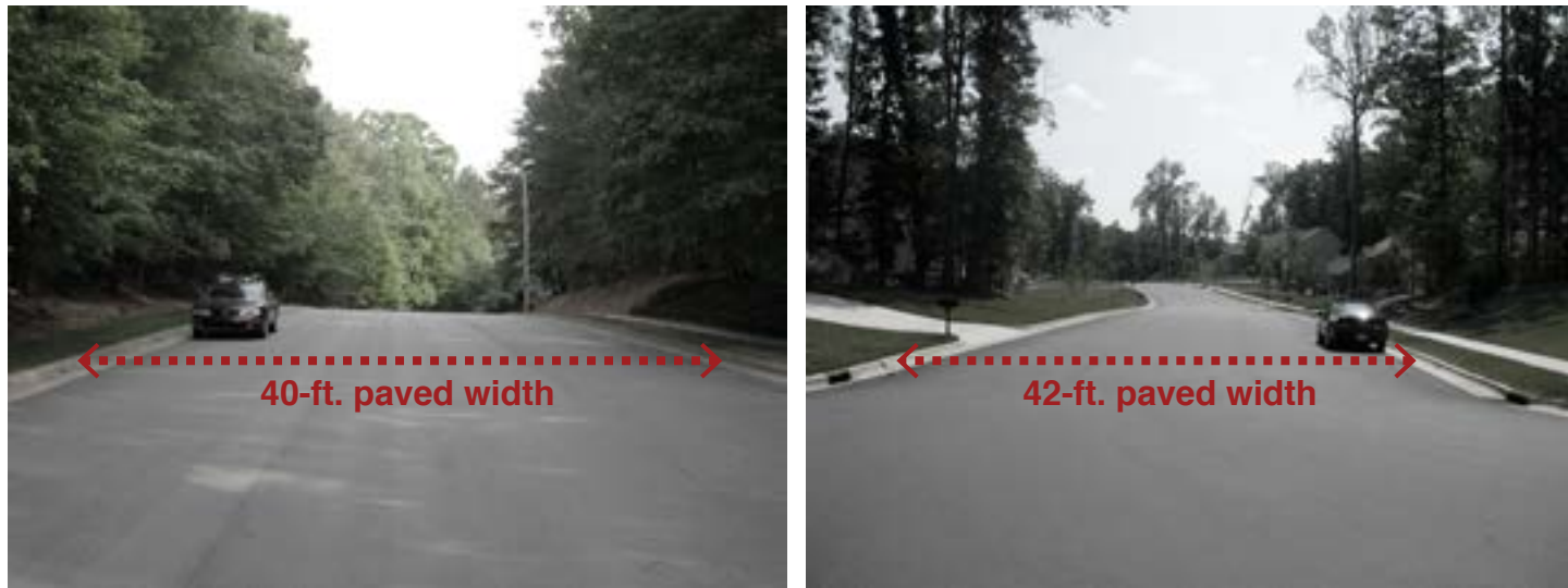
Figure 12: Residential Suburban Streets in Need of Retrofitting
