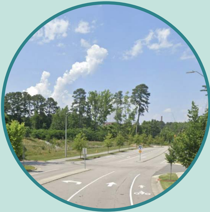
Pullen Road (separated lane)
