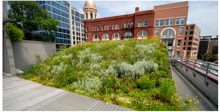
ASLA headquarters' green roof is one example of how landscape architects help reduce stormwater runoff while also conserving energy and improving air quality. Photo: ASLA
