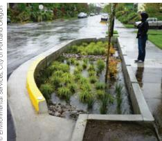
The City of Portland, OR has been a leader in incorporating green infrastructure practices into its water management. This curb cut rain garden allows runoff from the street to flow into a rain garden where it can slowly infiltrate into the ground, rather than flowing directly into the storm sewer.
