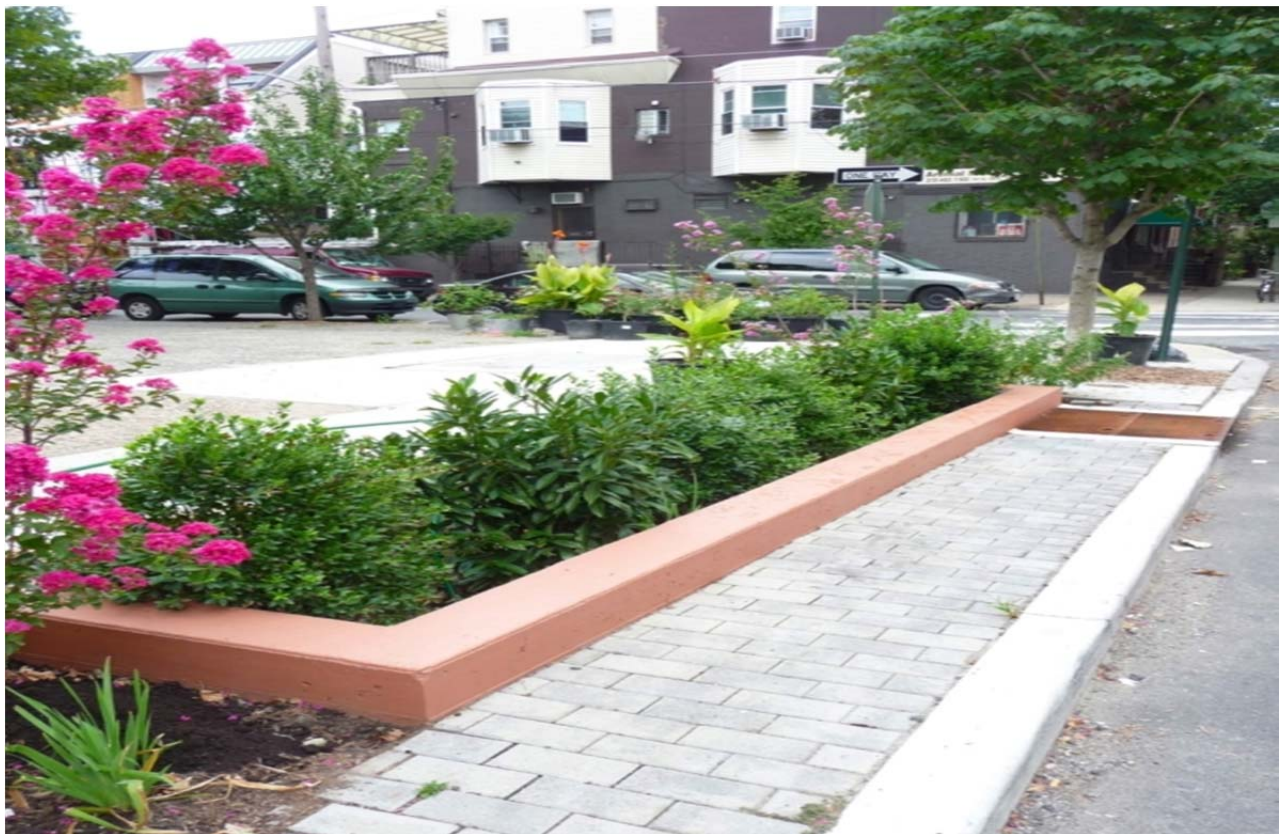
Photo Credit: Philadelphia Water Department
