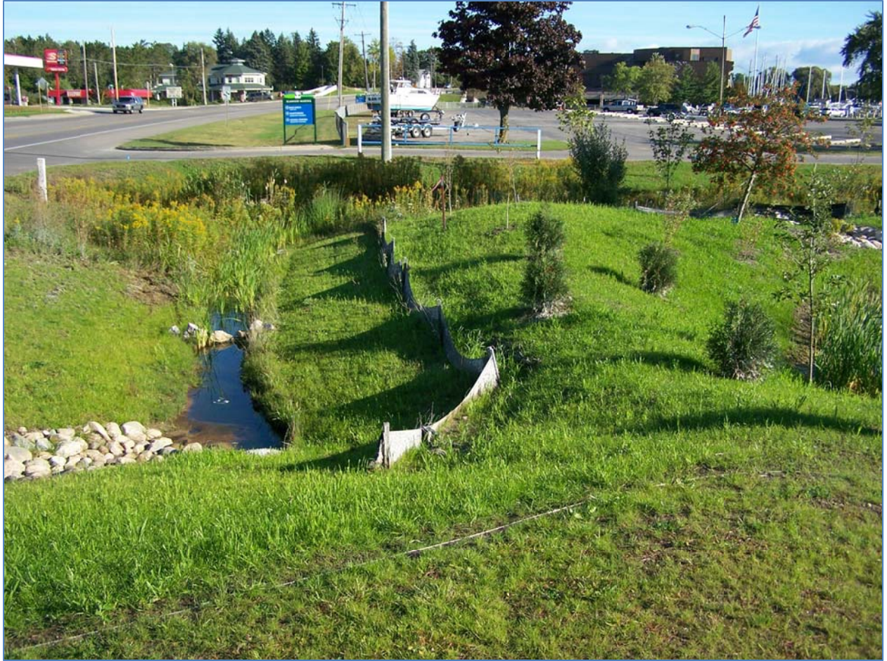
Photo: Gosling Czubak Engineering Sciences, Inc.
