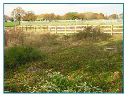
When a large storm or repeated storms occur the surge flows into leaching pools at the perimeter of the area and recharges on-site.
