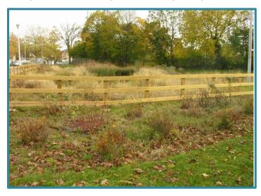
drainage for the field was reconfigured to provide a system that collected and detained the flow in a wet meadow/rain garden area that was designed in the location of a nuisance flood area. The detention area was planted with tolerant native species that process stormwater improving water quality. The combination of water and vegetation also provides wildlife habitat. Storm flow is dissipated by evapotranspiration, and ultimately is recharged on-site through leaching
