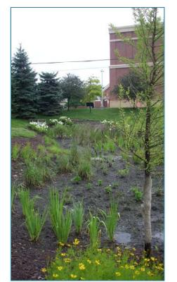
site infiltration. The 1,000 cubic foot detention basin was then planted with perennials, shrubs and ornamental grasses to create the rain garden. In addition to reducing stormwater runoff from the combined sewer system, the installation serves as an educational, green demonstration project.
