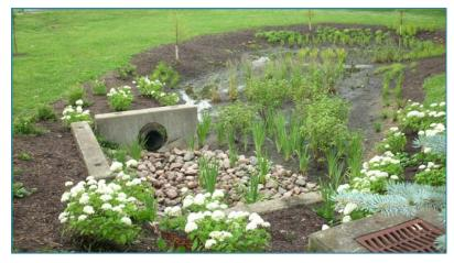
rain garden that captures and slowly releases stormwater runoff through on-site percolation or a slow release overflow structure.
