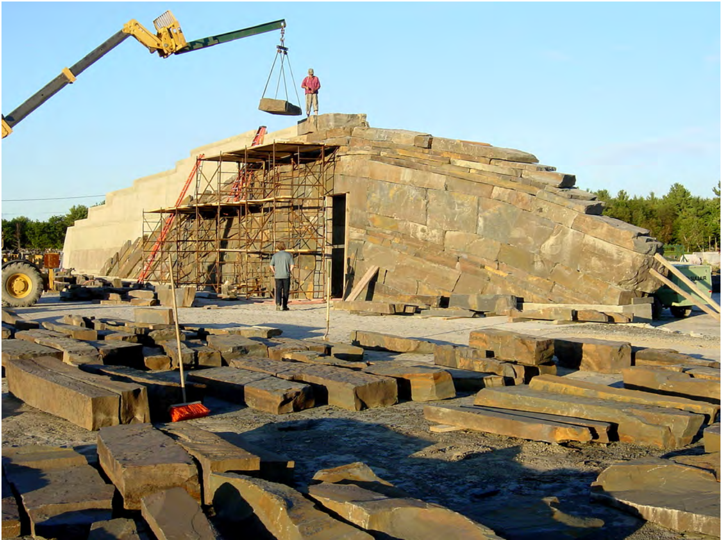
The bluestone ice wall mock-up for Teardrop Park at New York State Quarries in Alcove, NY
