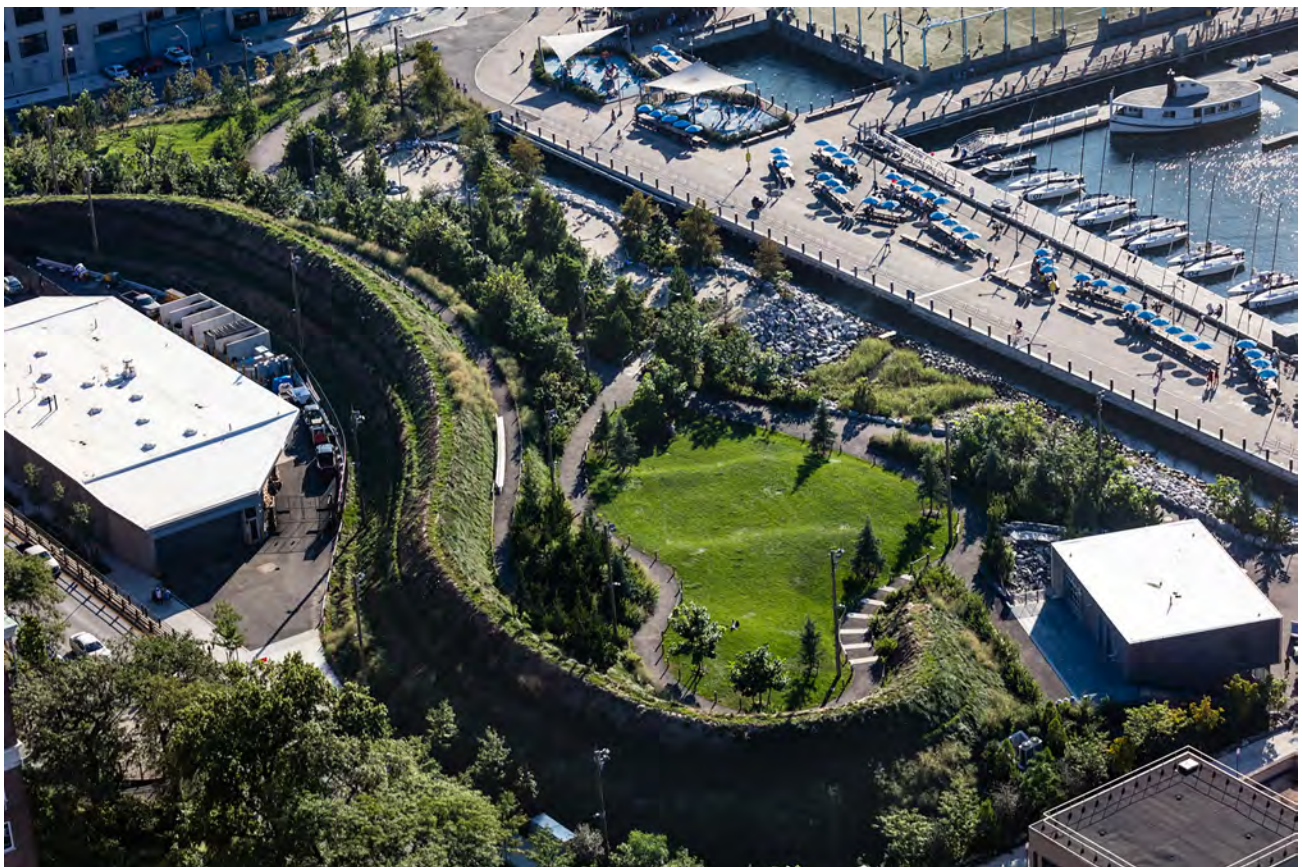
Construction of the sound berm at Brooklyn Bridge Park, a feat of engineering that shelters the park from the noise of the Brooklyn-Queens Expressway.
