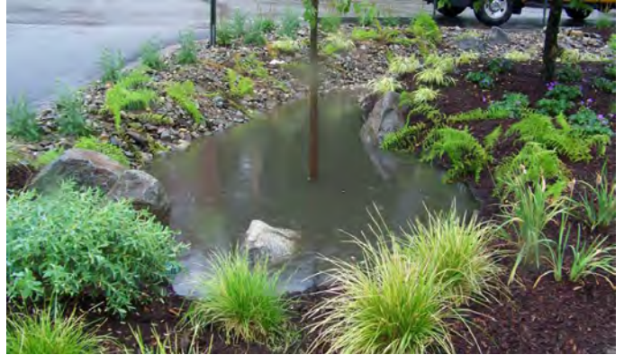
Landscape architects design green infrastructure like this rain garden at the Exeter Public Library that filters stormwater from the adjacent roadway and parking lot.
