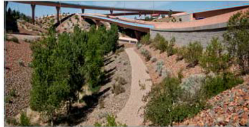
plantings, slope stabilization, and stormwater detention basins
