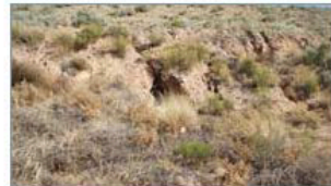
Before: erosion and weed proliferation
