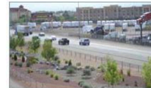
planted medians provide relief to drivers in an industrial corridor
