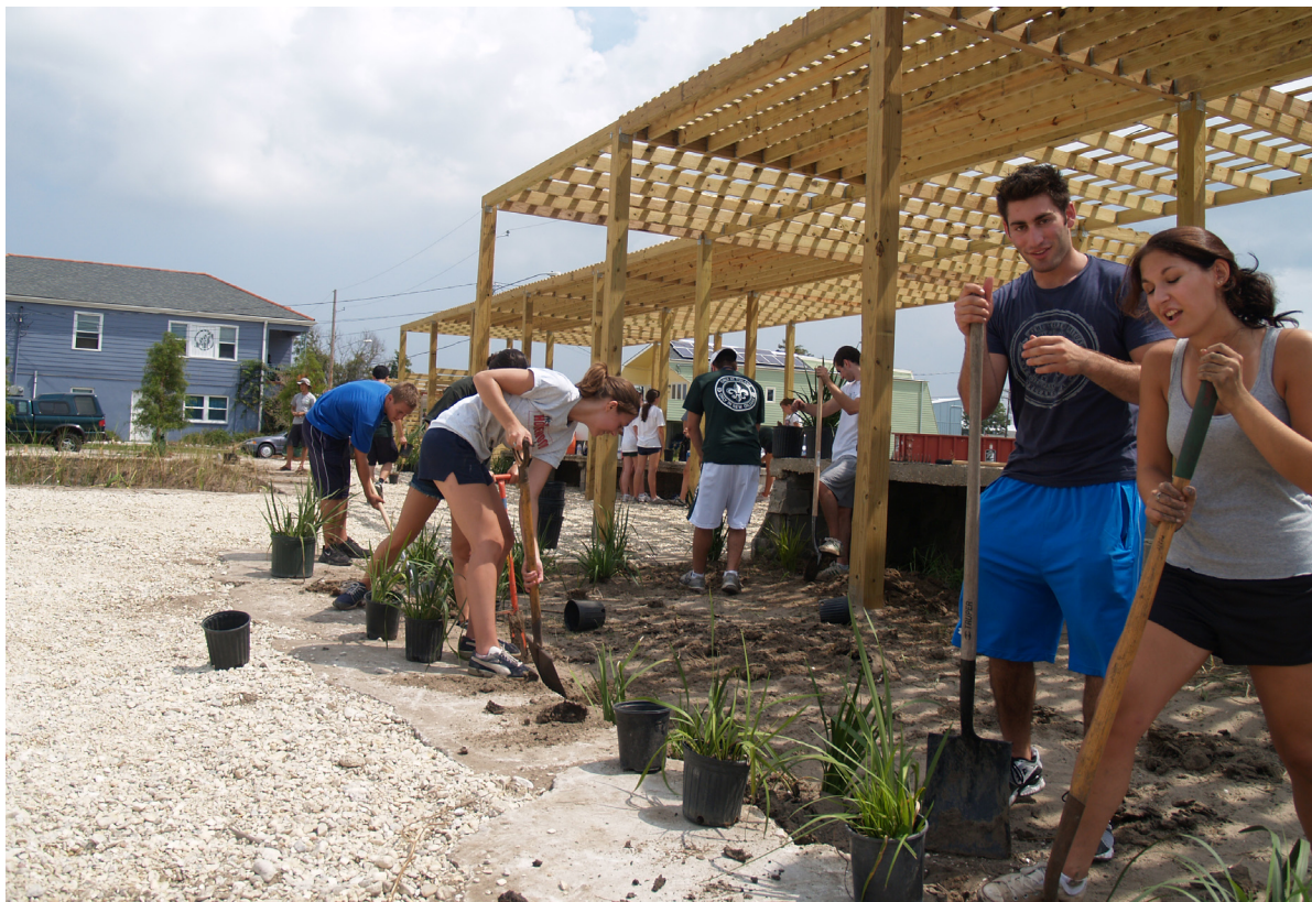
Volunteer installation of rain gardens at Pam's Place
