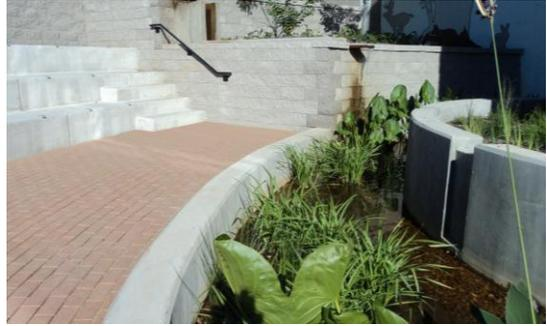
A permanently wet aquatic pool serves as the central focus of the outdoor classroom. Rain water is channeled through the aquatic pool and stormwater planters, from roof drains and the surrounding site, through a series of cascading rills above the pool. In this regard, the dynamics of rain events become a showcase that students may observe from the relative comfort of a glass enclosed staircase in the addition.
