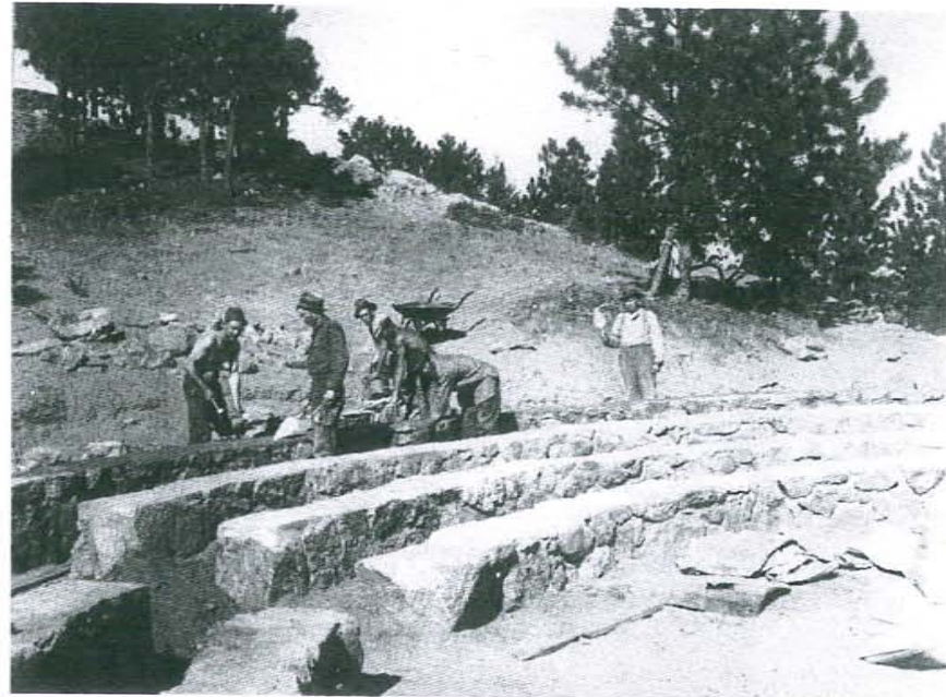
FIGURE 5. Enrollees mortar local stone at Flagstaff (NA).
