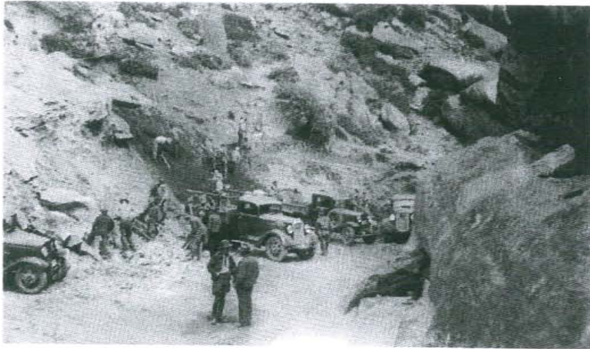
FIGURE 13. May–July 1936. Before the theatre was designed, enrollees built the stage, first cutting and filling the area around stage rock by hand (NA).
