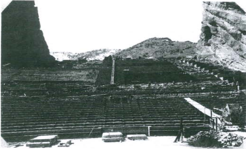
FIGURE 24. 1938. Looking up from the stage, one can again see how the enrollees built seats out from the middle and the stairs out from the ledge to meet each other. Note the gap of unpoured rows in the upper righthand corner of the theatre (DPL).
