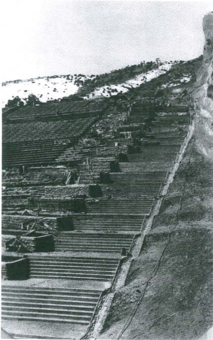
FIGURE 22. 1938. To mesh the theatre and the newly revealed ledge, enrollees did not pour the seats all the way out to the northern edge until the north stair and planters were built bugging the exposed ledge of Creation Rock. Seating was built from the middle (left to right in the photograph) and the stair out from the rock wall (right to left) to eventually meet. The stair planters were similarly test built to fit (DPL).
