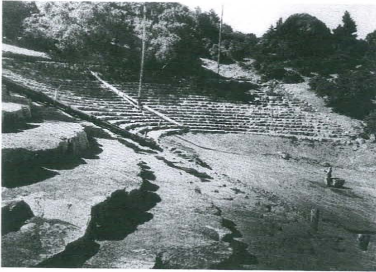
FIGURE 42. c. 1937–1938. Upon completion of the lower 20 rows, the 80-foot high booms were relocated to the top of the theatre and a track rail was installed along the middle aisle to distribute stone across the site more quickly (UCCEDA).
