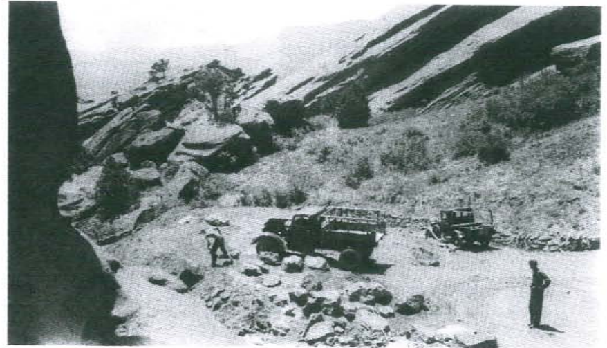
FIGURE 14. 1936. The CCC recruits seldom had access to heavy earthmoving equipment but instead relied on the limited mechanical resources shown in these photos. (NA).
