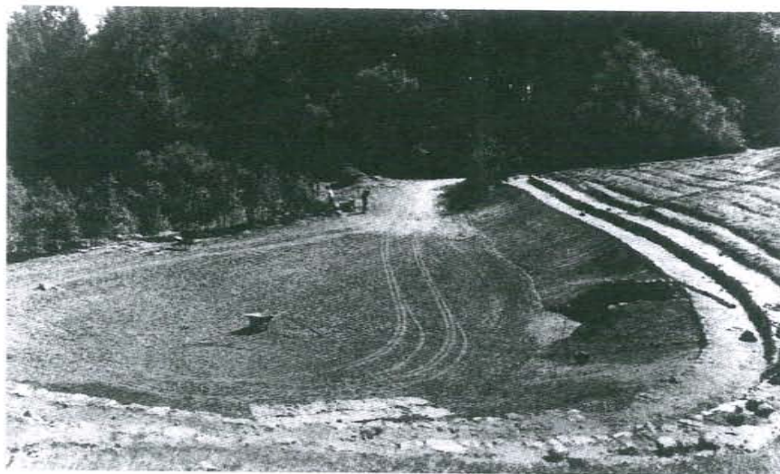
FIGURE 36. A screen of chicaquin oaks was planted as a backdrop to the stage. The embankment between the stage and auditorium was high enough to accommodate the prompter's box shown above (NA).
