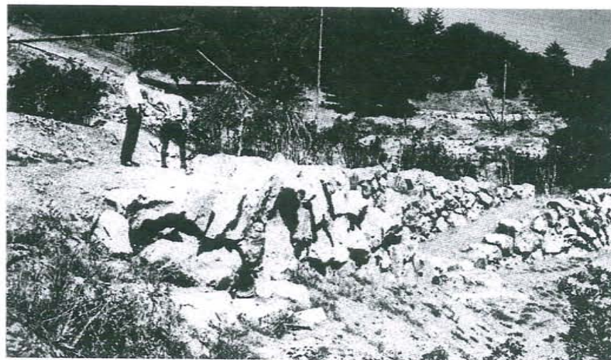
FIGURE 37. Stone retaining walls supported the 12 feet of fill in the ravine that once crossed the stage. These walls also allowed actors to move from stage left to stage right without being seen (MHS).
