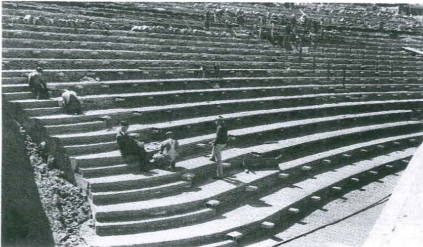
FIGURE 25. 1938. The contrast between the sandstone face of the risers and the bright, smooth concrete of the aisles was an onsite decision made in response to an observation by a traveling CCC inspector (DPL).
