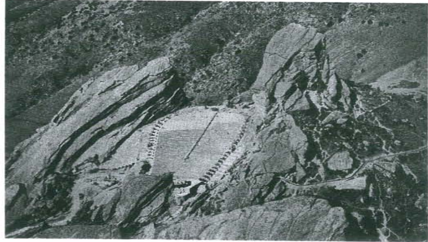
FIGURE 26. 1941. An aerial view taken just before completion shows the construction conveyor still in place down the centre of the theatre highlighting the final asymmetrical form and illustrating how it reflects the distinct gestures of the two rock walls ( The American City , March 1944).
