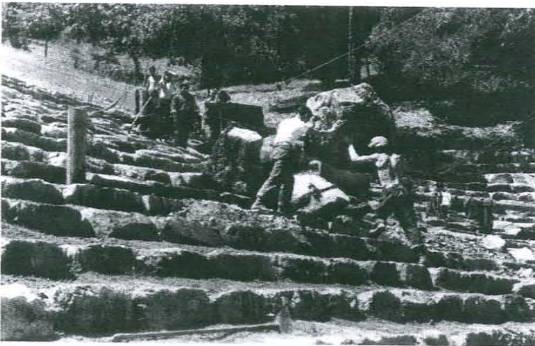
FIGURE 43. 1937. Per Knight's instructions, workers selected stones with two surfaces at right angles to provide a flat top and vertical riser without compromising the weathered look of the stones by cutting them (NA).
